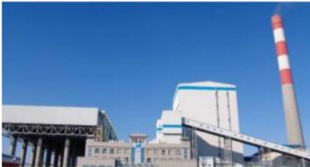
17.7 MW 35kV Project for Ningxia Dianjian Shenhua Lingwu
