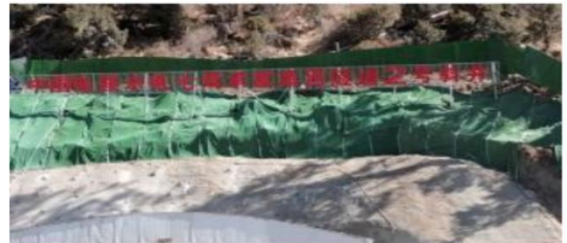
China Electric Power Construction Seventh Bureau Moxi Tunnel 2# inclined shaft
