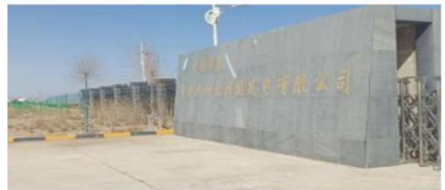
Huarun Power Yuanyang 35MW Distributed Wind Power Project
