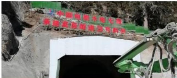
China Electric Power Construction Seventh Bureau Moxi Tunnel 3# inclined shaft
